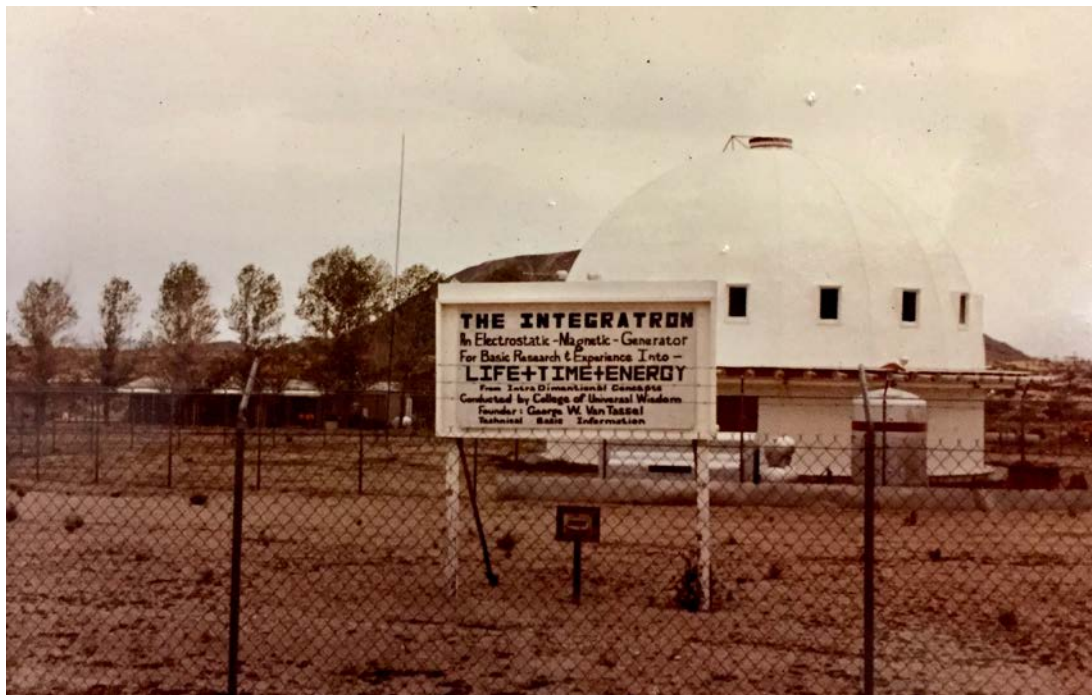
Figure 32. 35mm image of Integratron, ca. 1977. Machinery visible in front of structure was removed immediately after George Van Tassel's passing. View: E.
